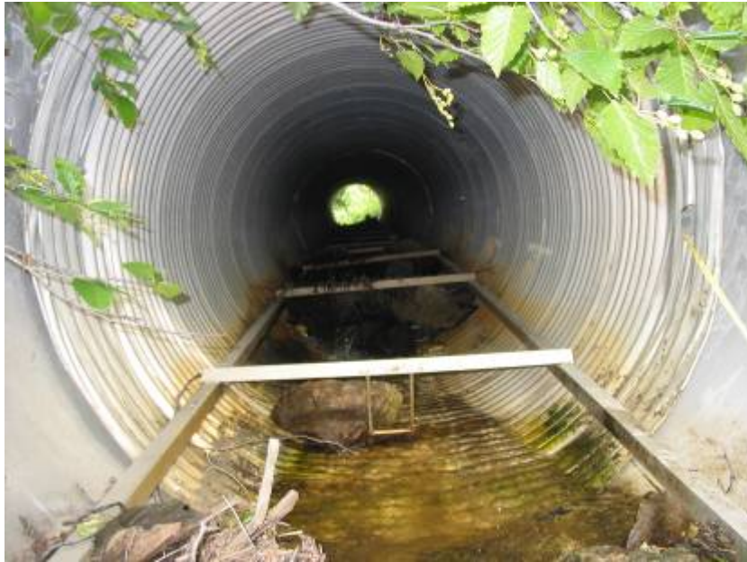
Figure 4. Metal detachable fishway.
