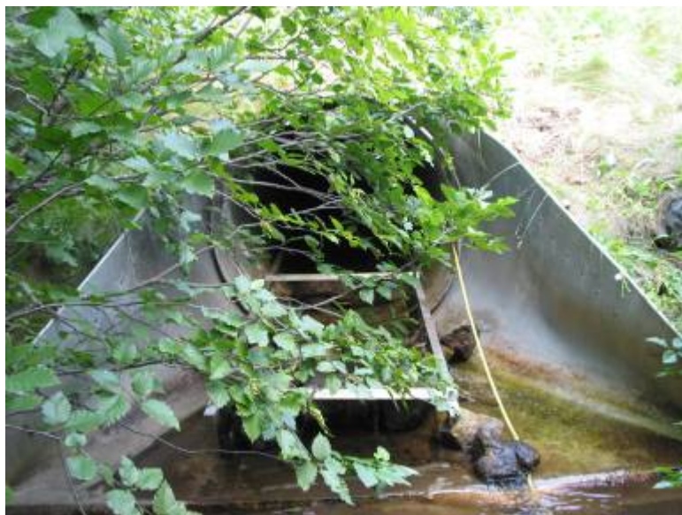
Figure 3. Existing culvert outfall at Holgate Creek below Mud Bay Road.
