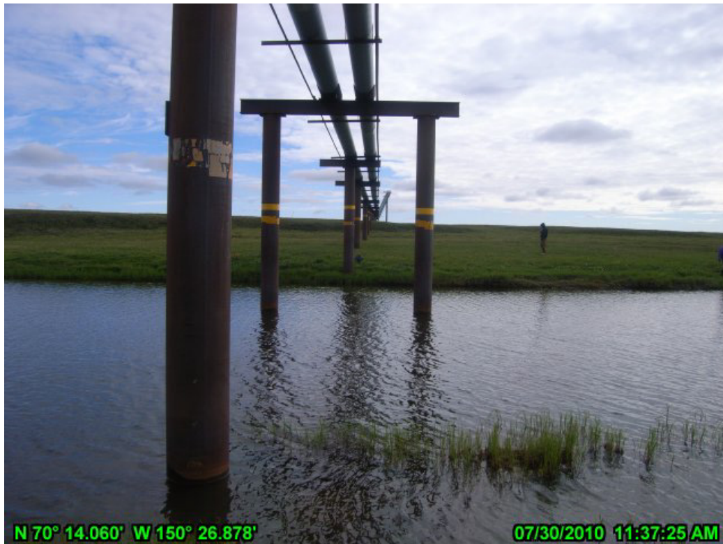
PHOTO A.17 KACHEMACH RIVER CROSSING, JULY 30, 2010: WEST BANK LOOKING EAST
