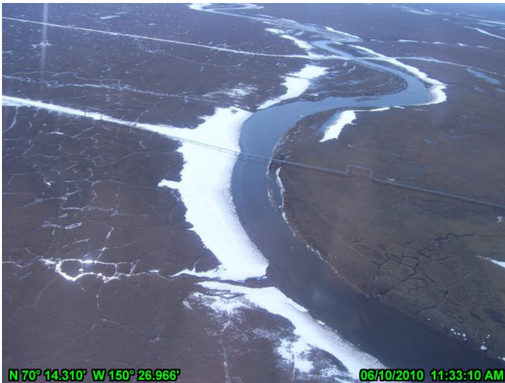
PHOTO A.14 KACHEMACH RIVER CROSSING, JUNE 10, 2010: LOOKING SOUTHEAST
