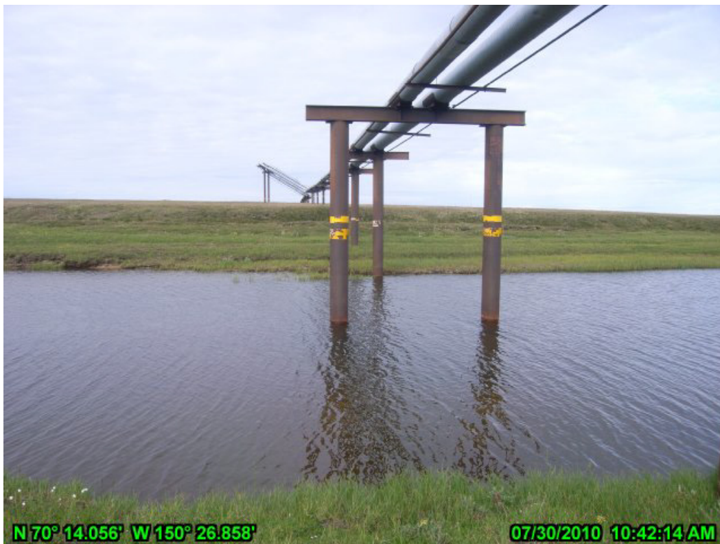
PHOTO A.18 KACHEMACH RIVER CROSSING, JULY 30, 2010: EAST BANK LOOKING WEST
