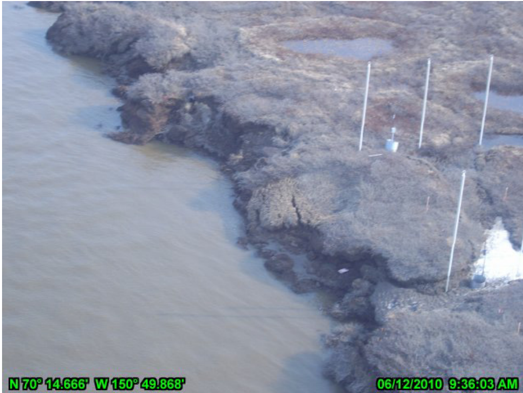
PHOTO A.9 HDD EAST, JUNE 12, 2010: CLOSE-UP EAST BANK, LOOKING NORTHEAST
