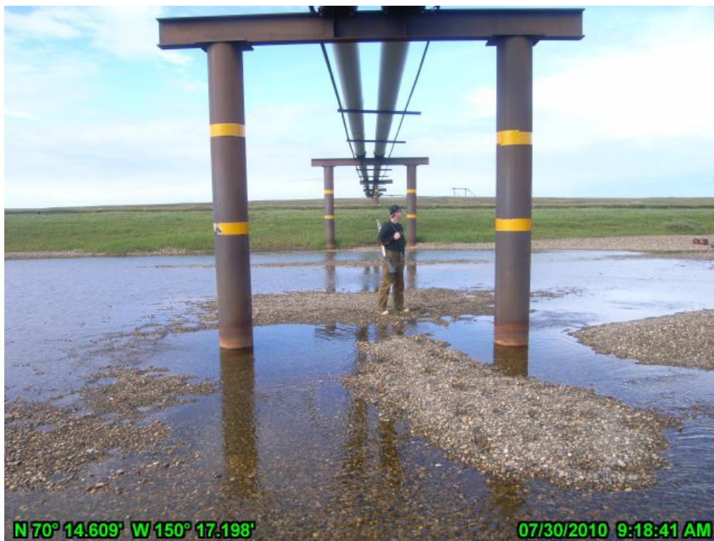
PHOTO A.28 MILUVEACH RIVER CROSSING, JULY 30, 2010: EAST BANK, LOOKING WEST
