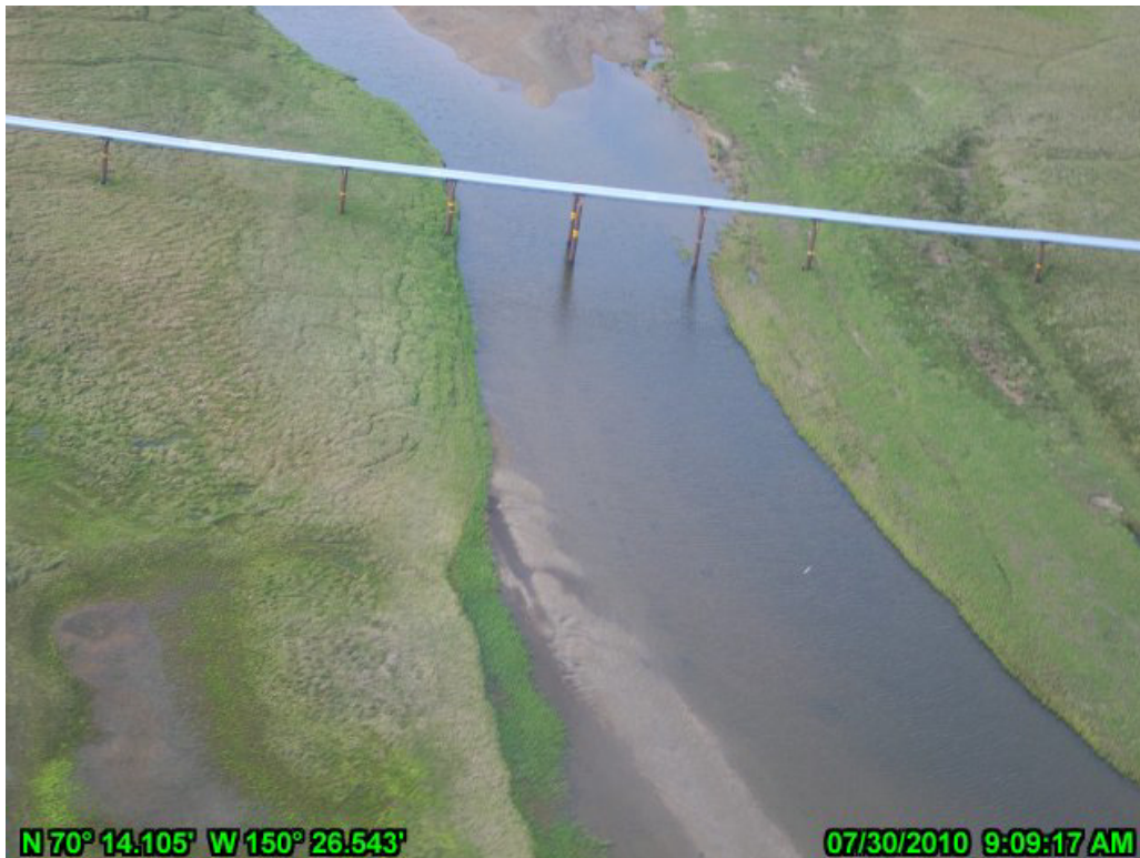
PHOTO A.16 KACHEMACH RIVER CROSSING, JULY 30, 2010: LOOKING SOUTH
