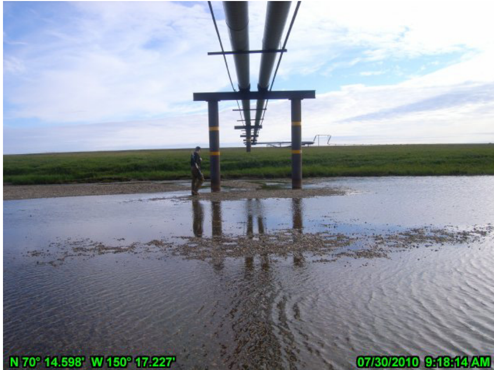
PHOTO A.27 MILUVEACH RIVER CROSSING, JULY 30, 2010: WEST BANK, LOOKING EAST
