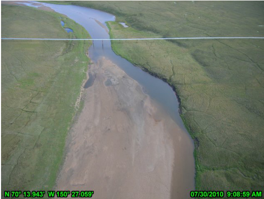
PHOTO A.15 KACHEMACH RIVER CROSSING, JULY 30, 2010: LOOKING NORTH
