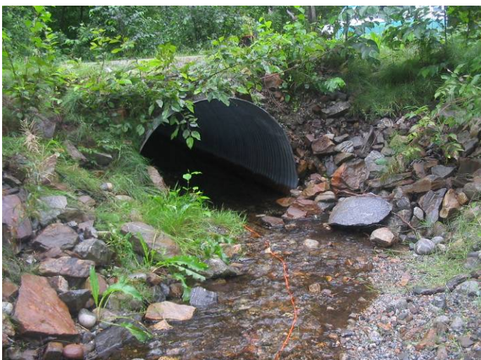
Reach 2 - Culvert under Liarsville Road. View looking downstream.
