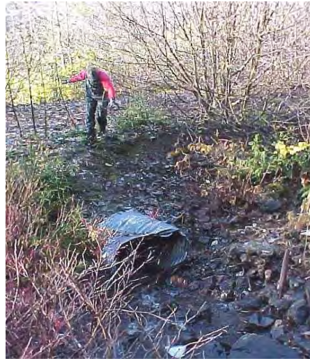
Photo 35 and 36. Non-functional culverts upper Arrow Creek, reach A2.
