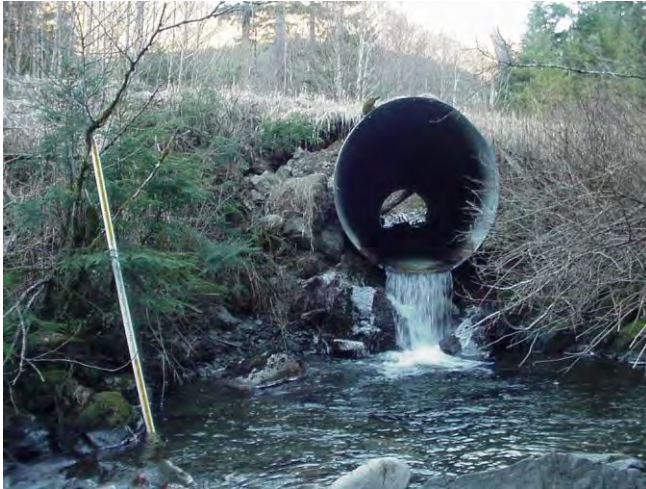
Photo 34. 7-mile Creek culvert along Klawock Hollis Highway Crossing.
