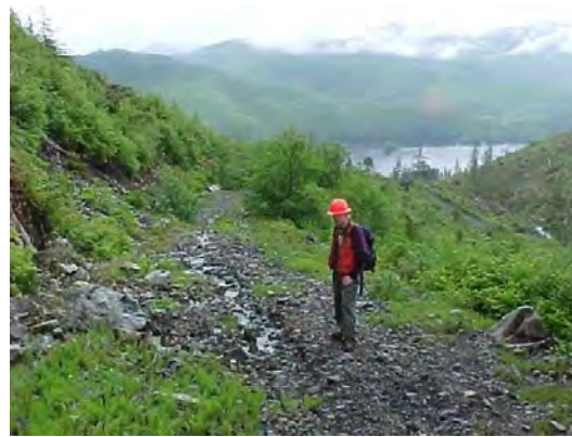
Photo 37. Landslides visible from Upper Bluewater Creek. Photo 38. Water on road surface from failed cross drain, upper Bluewater road system.
