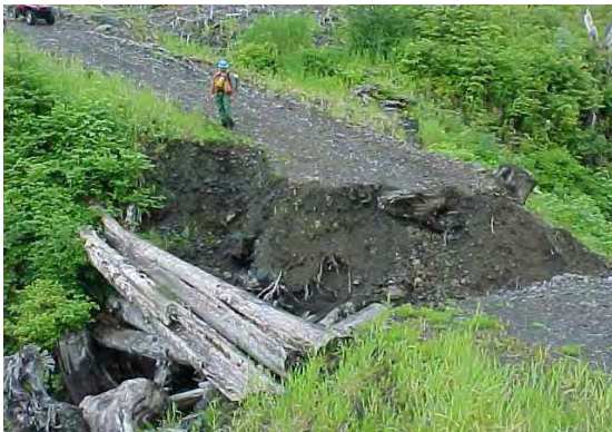
Photo 32. Blown stream crossing on small stream draining in to Trib 2 upper Hatchery Creek. Photo 33. Hatchery Creek, reach HT2C.
