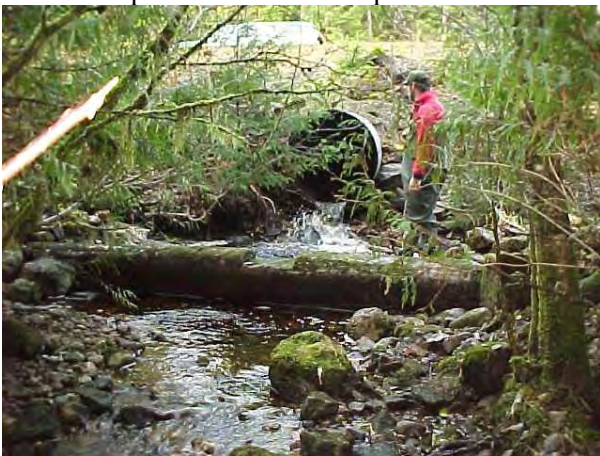
Photo 19. Reach KT5 (Trib 5) below highway crossing.
