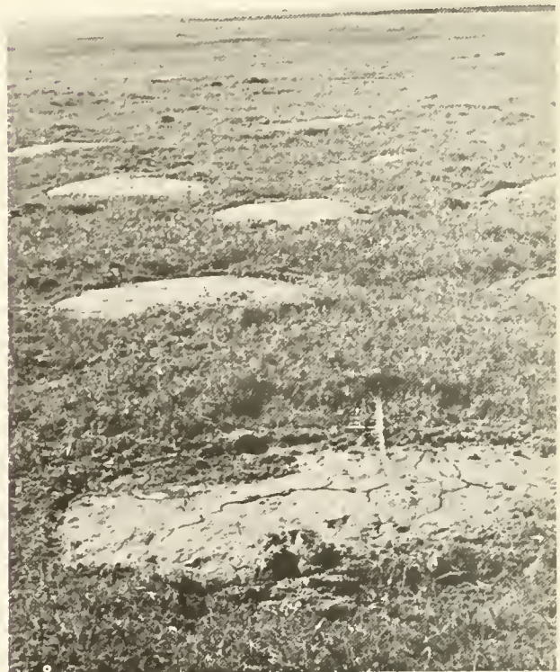
Type 8 vegetation of active frost boils with little vegetation as a result of disturbance by road construction equipment.
