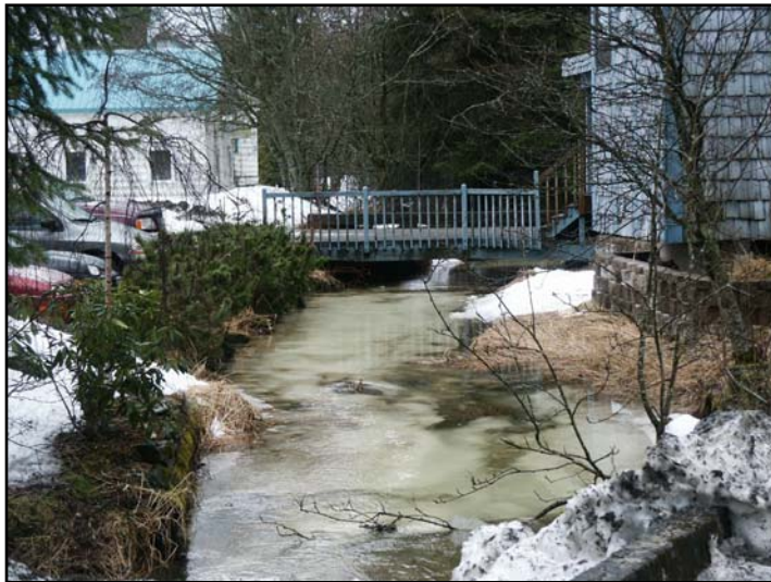
Figure 14: Buildings and parking areas in lower Jordan Creek that are situated within the 50-foot setback. February, 2004.
