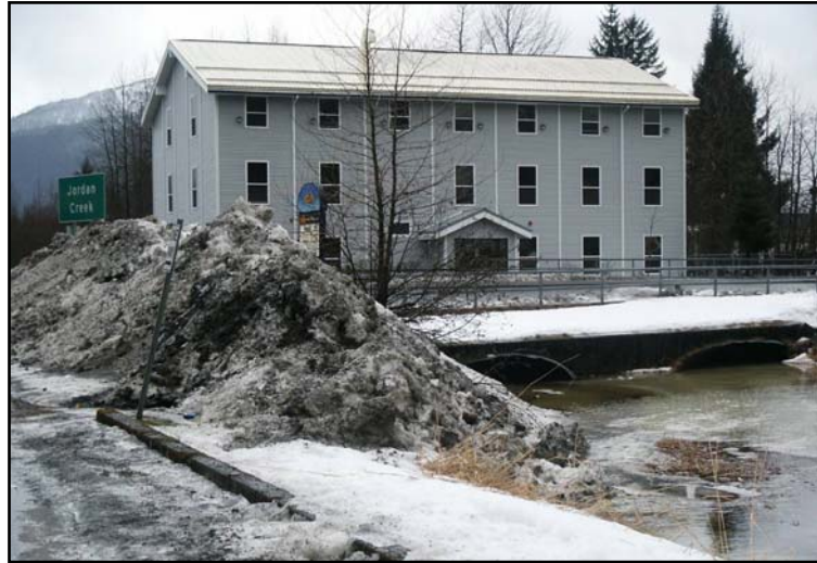
Figure 8: Snow plowed from streets and driveways stored in the creek near Jordan Creek Center. Sediment and debris are deposited in the creek when the snow melts. February, 2005.
