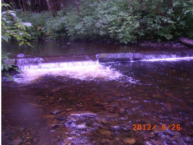
Figure 4. A structure put in place by ADF&G in 1992 to function as a sill log. Although this structure has created a pool directly below the structure, the channel has remained mostly uniform both upstream and downstream from the structure.
