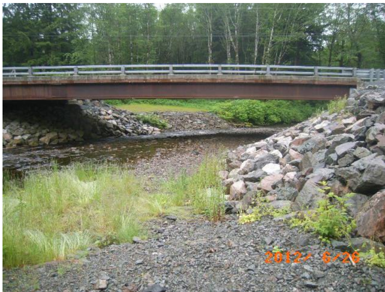
Figure 5. Looking downstream at the new bridge and unvegetated banks.
