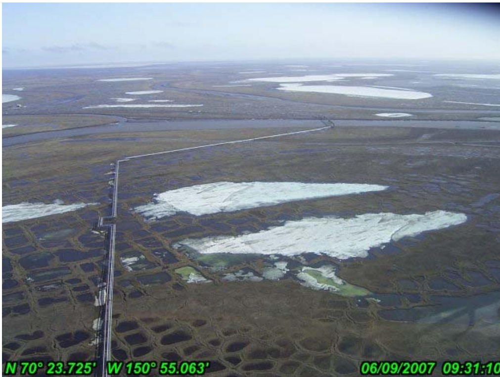
Photo 20 L9907 (top) south of Ulam Channel pipeline crossing
