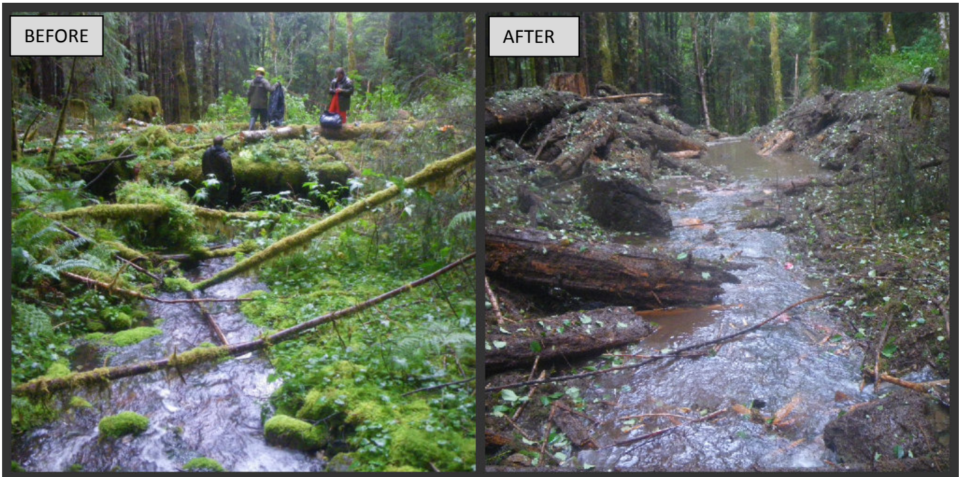
Photo set 5 – Road decommissioning before and after treatment.
