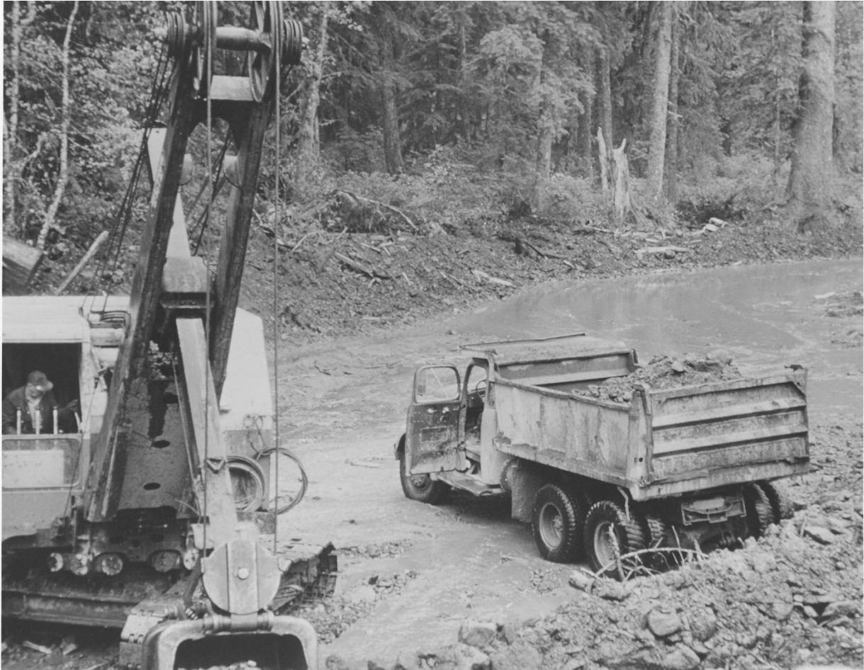
Twelvemile Creek during road building and timber harvest in 1960.
