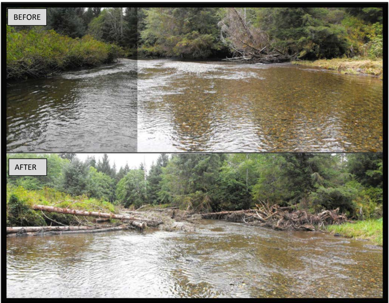
Photo set 3 – Phase II, Structure Number 18, looking downstream before and after LW placement.
