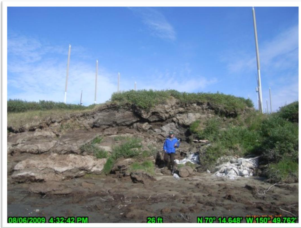
PHOTO A.9 HDD EAST, AUGUST 6, 2009. VIEW OF EAST BANK FROM CHANNEL.
