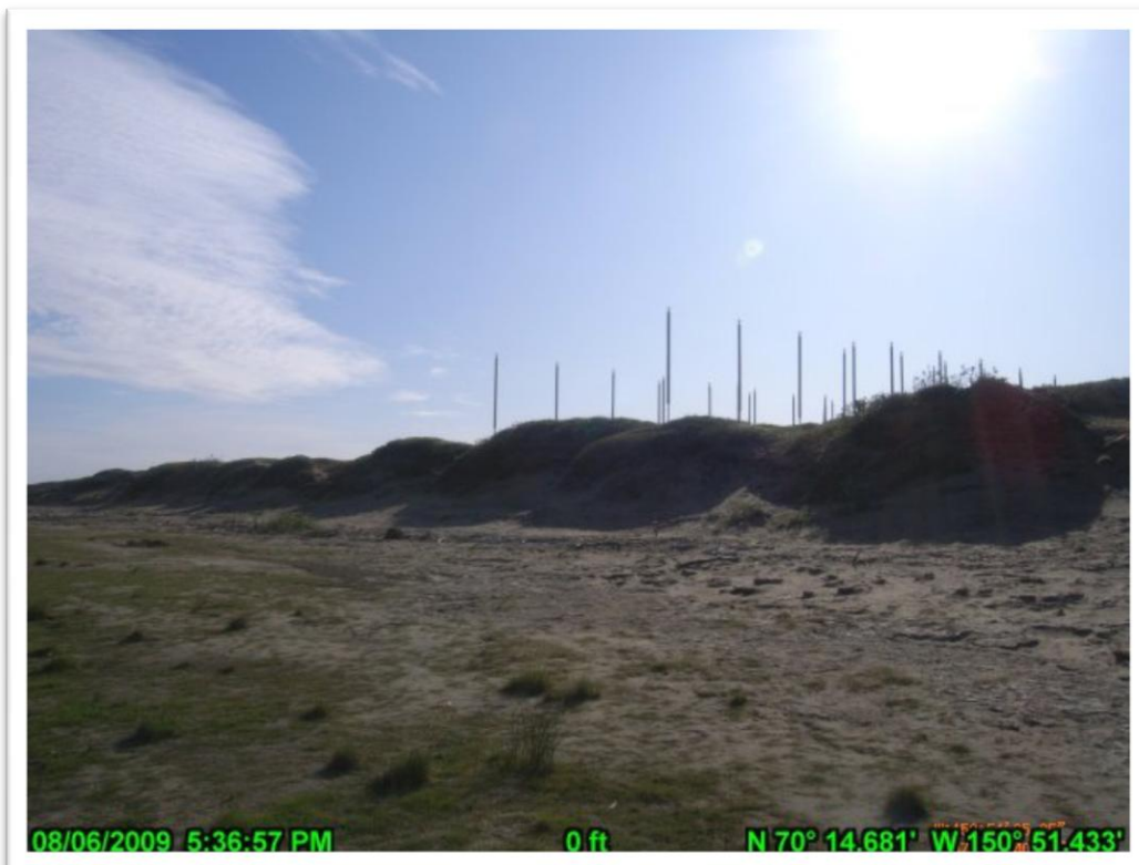
PHOTO A.4 HDD WEST, AUGUST 6, 2009. WEST BANK, LOOKING SOUTHWEST.
