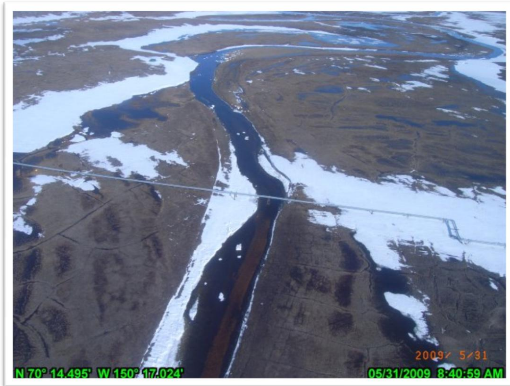
PHOTO A.23 MILUVEACH RIVER CROSSING, MAY 31, 2009. PIPE BRIDGE AT MILUVEACH RIVER CROSSING DURING SPRING BREAKUP.
