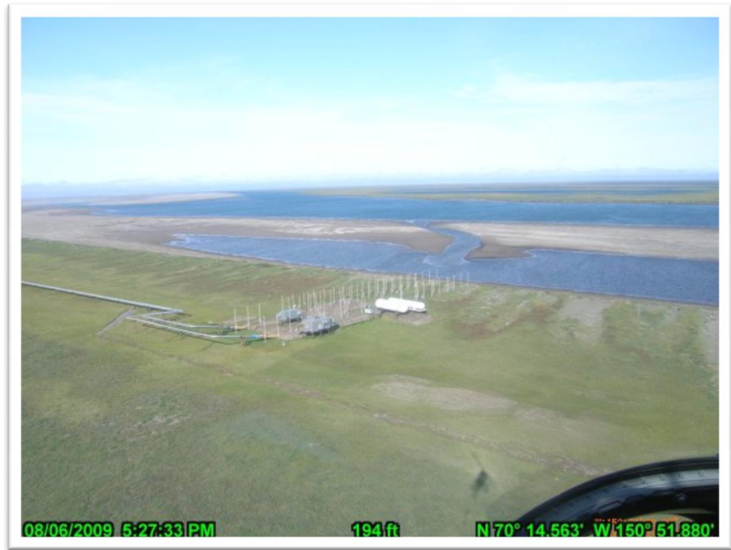
PHOTO A.2 HDD WEST, AUGUST 6, 2009. AERIAL VIEW OF HDD WEST FACILITIES.
