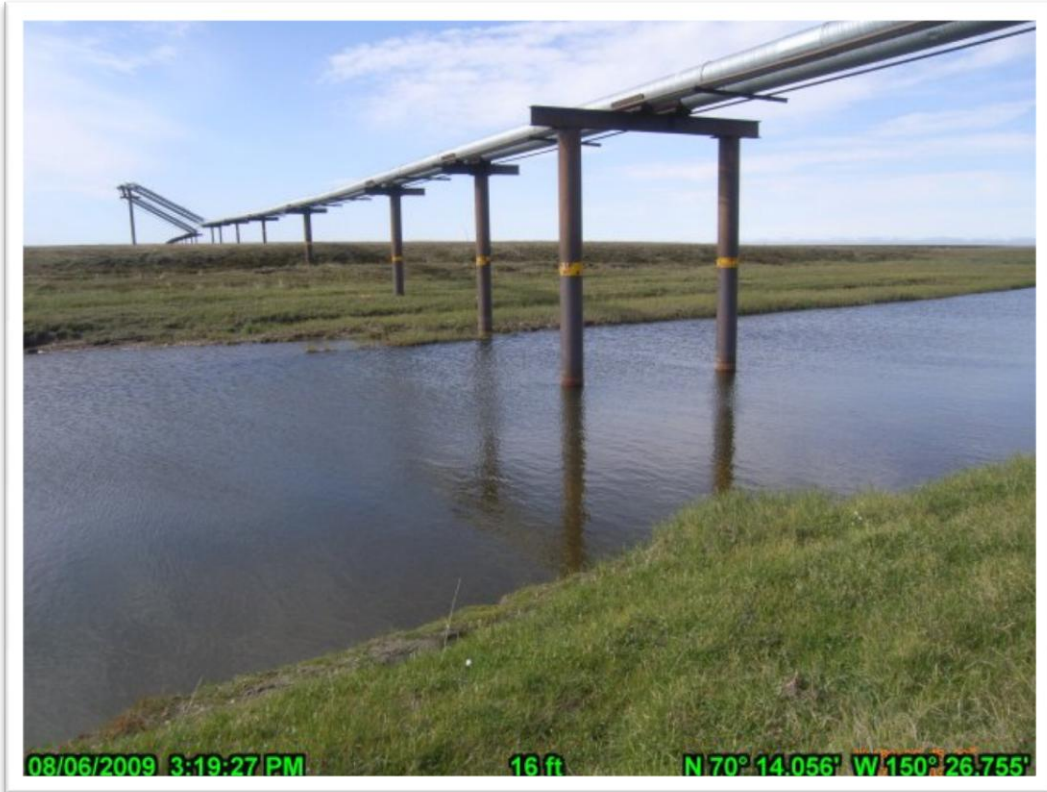
PHOTO A.21 KACHEMACH RIVER CROSSING, AUGUST 6, 2009. EAST BANK, LOOKING WEST.
