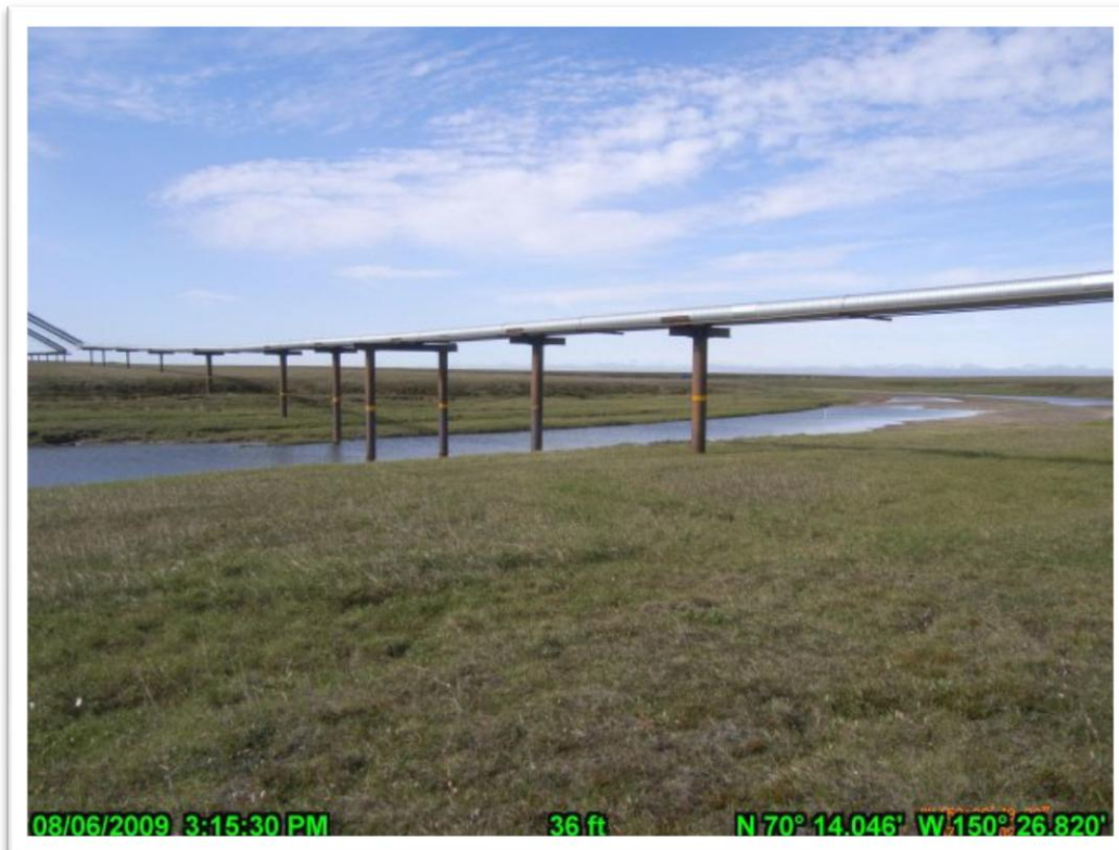
PHOTO A.20 KACHEMACH RIVER CROSSING, AUGUST 6, 2009. EAST BANK, LOOKING NORTHWEST.
