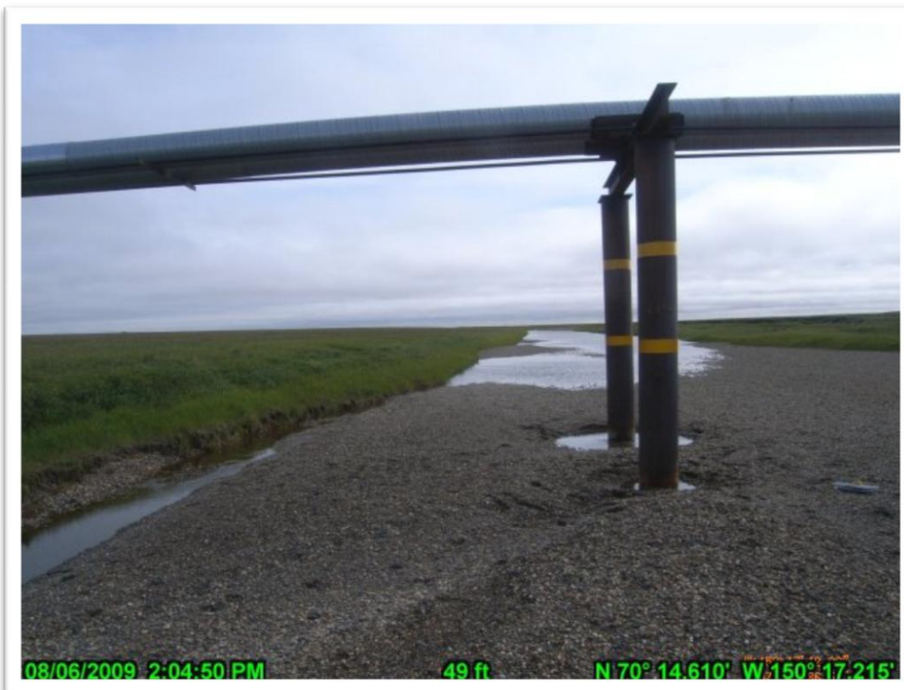
PHOTO A.26 MILUVEACH RIVER CROSSING, AUGUST 6, 2009. IN CHANNEL LOOKING SOUTH.
