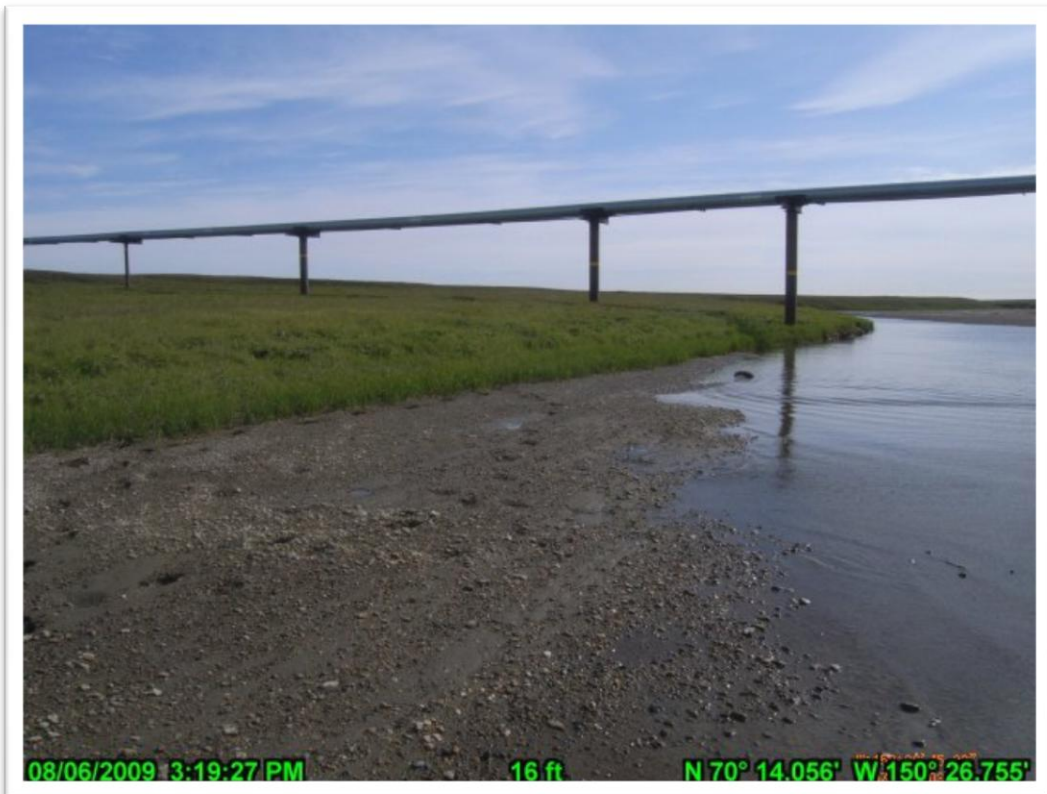
PHOTO A.22 KACHEMACH RIVER CROSSING, AUGUST 6, 2009. EAST BANK LOOKING SOUTH.
