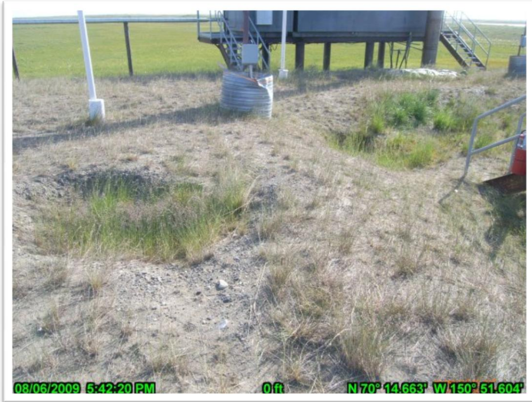
PHOTO A.5 HDD WEST, AUGUST 6, 2009. VIEW OF PITS IN GRAVEL PAD BETWEEN CP MODULE BUILDINGS.
