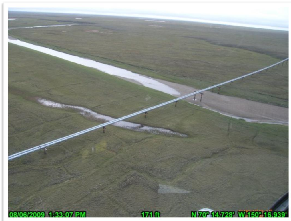
PHOTO A.24 MILUVEACH RIVER CROSSING, AUGUST 6, 2009. AERIAL VIEW OF CROSSING, LOOKING SOUTHWEST.
