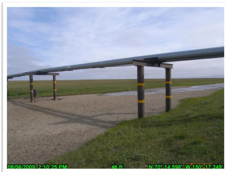
PHOTO A.28 MILUVEACH RIVER CROSSING, AUGUST 6, 2009. FROM WEST BANK LOOKING SOUTHEAST.
