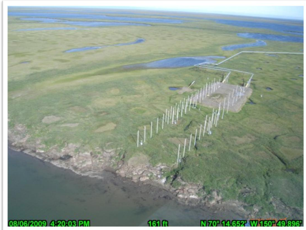
PHOTO A.8 HDD EAST, AUGUST 6, 2009. AERIAL VIEW OF HDD EAST, LOOKING EAST.
