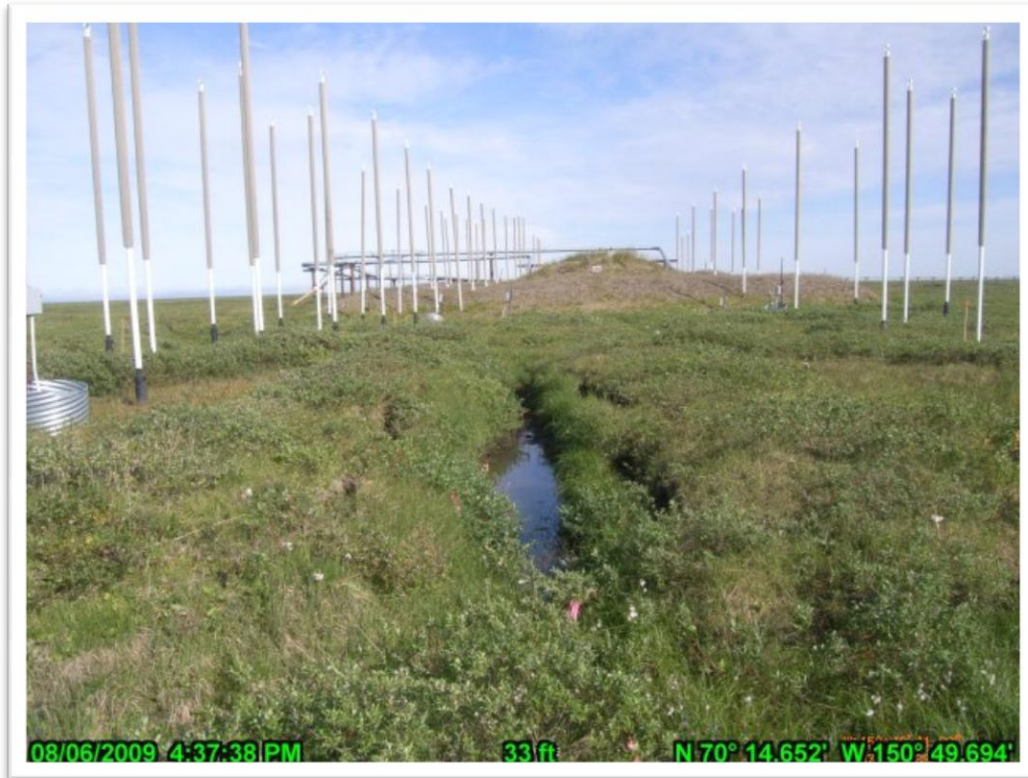
PHOTO A.11 HDD EAST, AUGUST 6, 2009. VIEW OF TROUGH FROM EAST BANK, LOOKING EAST TOWARD PIPELINE.
