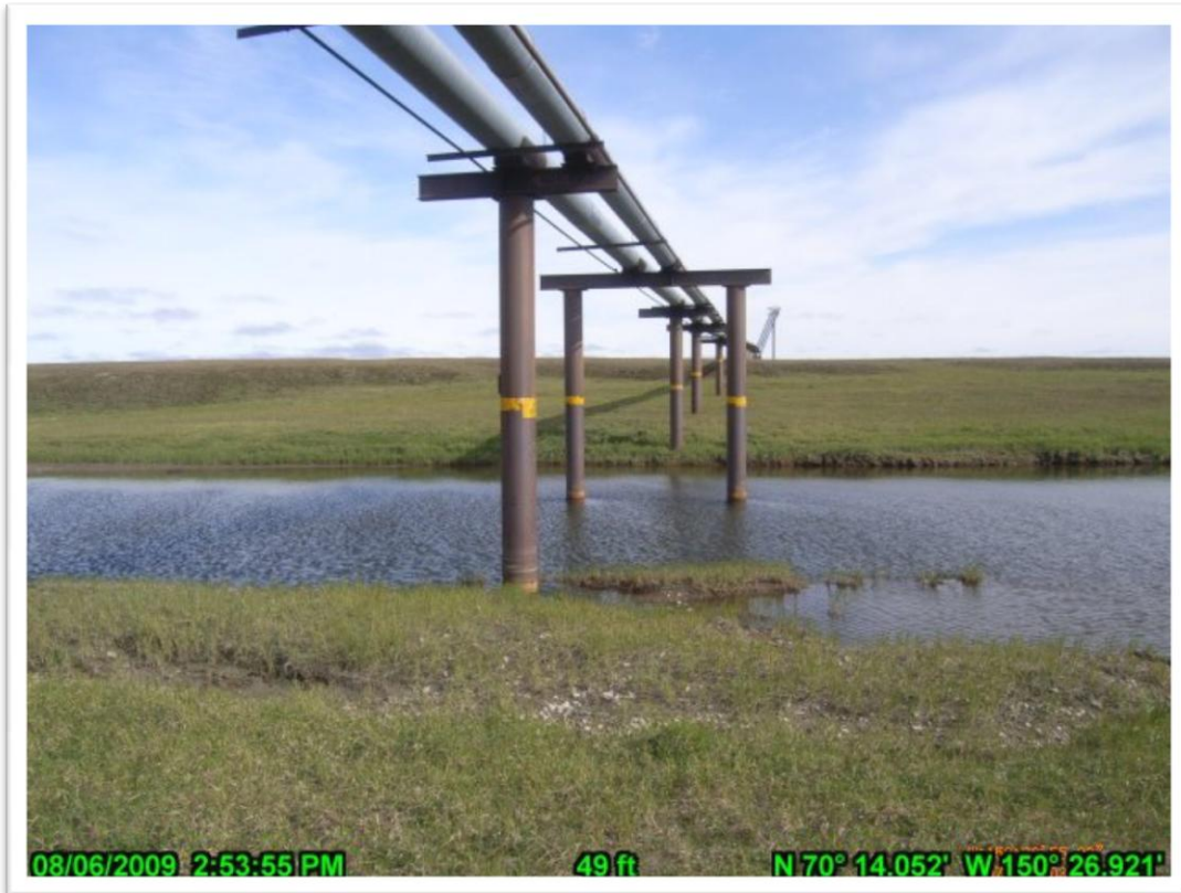
PHOTO A.17 KACHEMACH RIVER CROSSING, AUGUST 6, 2009. FROM WEST BANK, LOOKING EAST.
