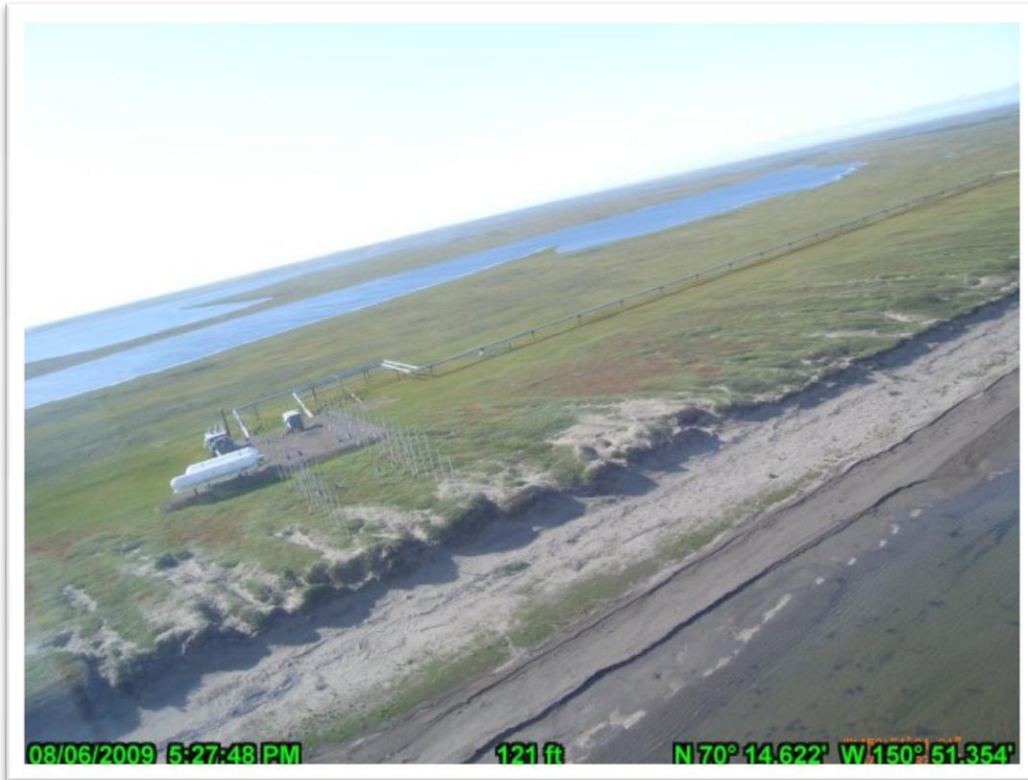
PHOTO A.3 HDD WEST, AUGUST 6, 2009. WEST BANK, LOOKING NORTHWEST.
