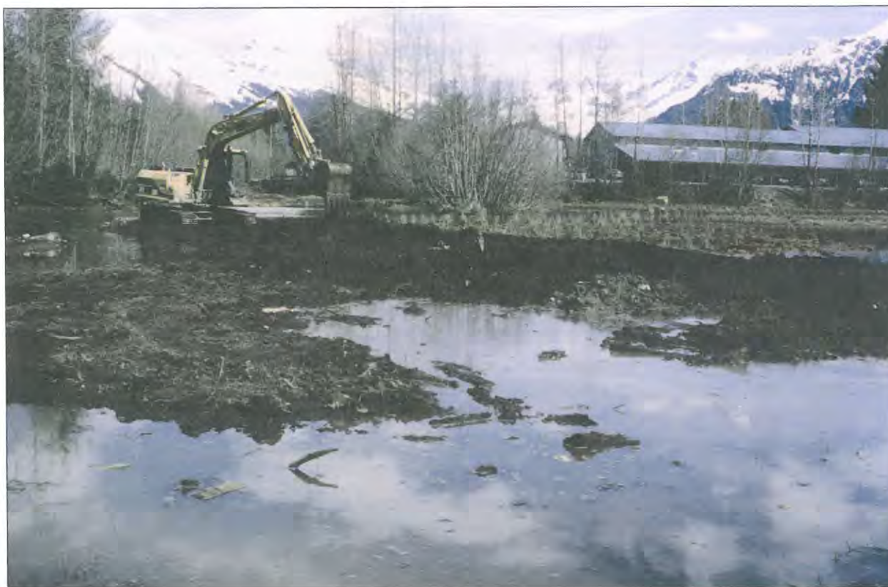
Figure 12.--The dredge pond that was developed into a stormwater treatment marsh. (Photo by NMFS).
