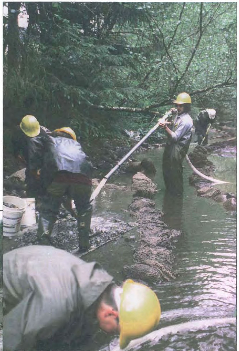
Figure 10.--An Americorps crew using dredging equipment to remove fine sediment from a salmon spawning area in Duck Creek. (Photo by NMFS).
