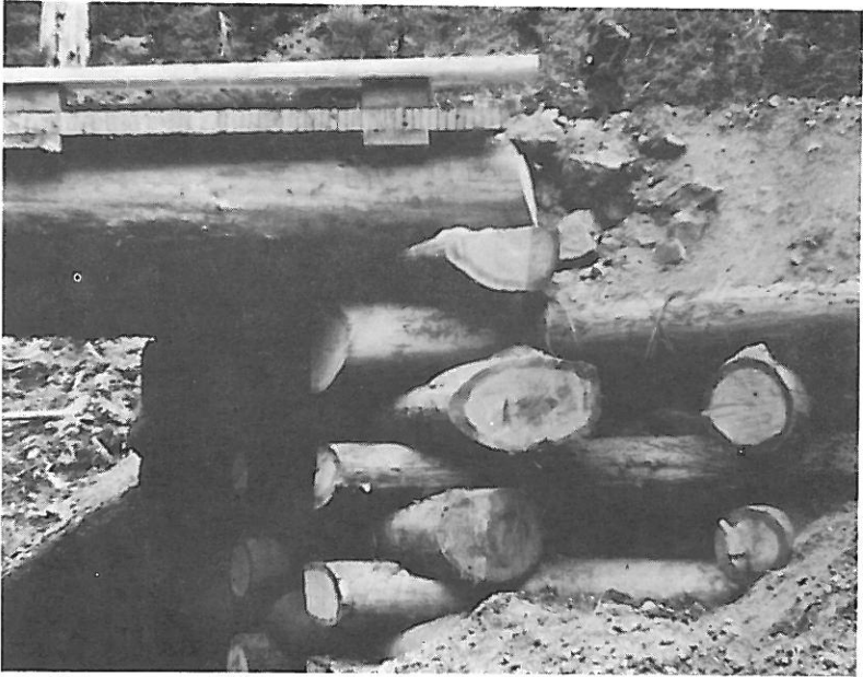
Figure 18.--This is a properly constructed crib retaining wall.
